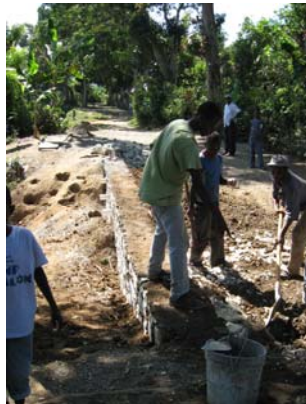
Retaining wall with drain-pipe, on the road.
