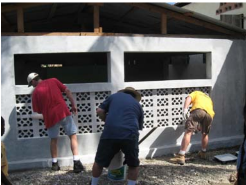
Starting to paint the school.
