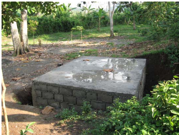
The septic tank is finished!
