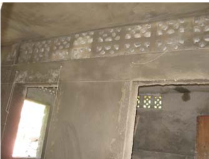
Wall finishing in kitchen depot.
