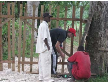
John working on the gate.
